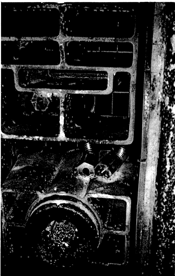
Figure 13—Corner Burners with Fiber Optic Scanners Welded in Place
